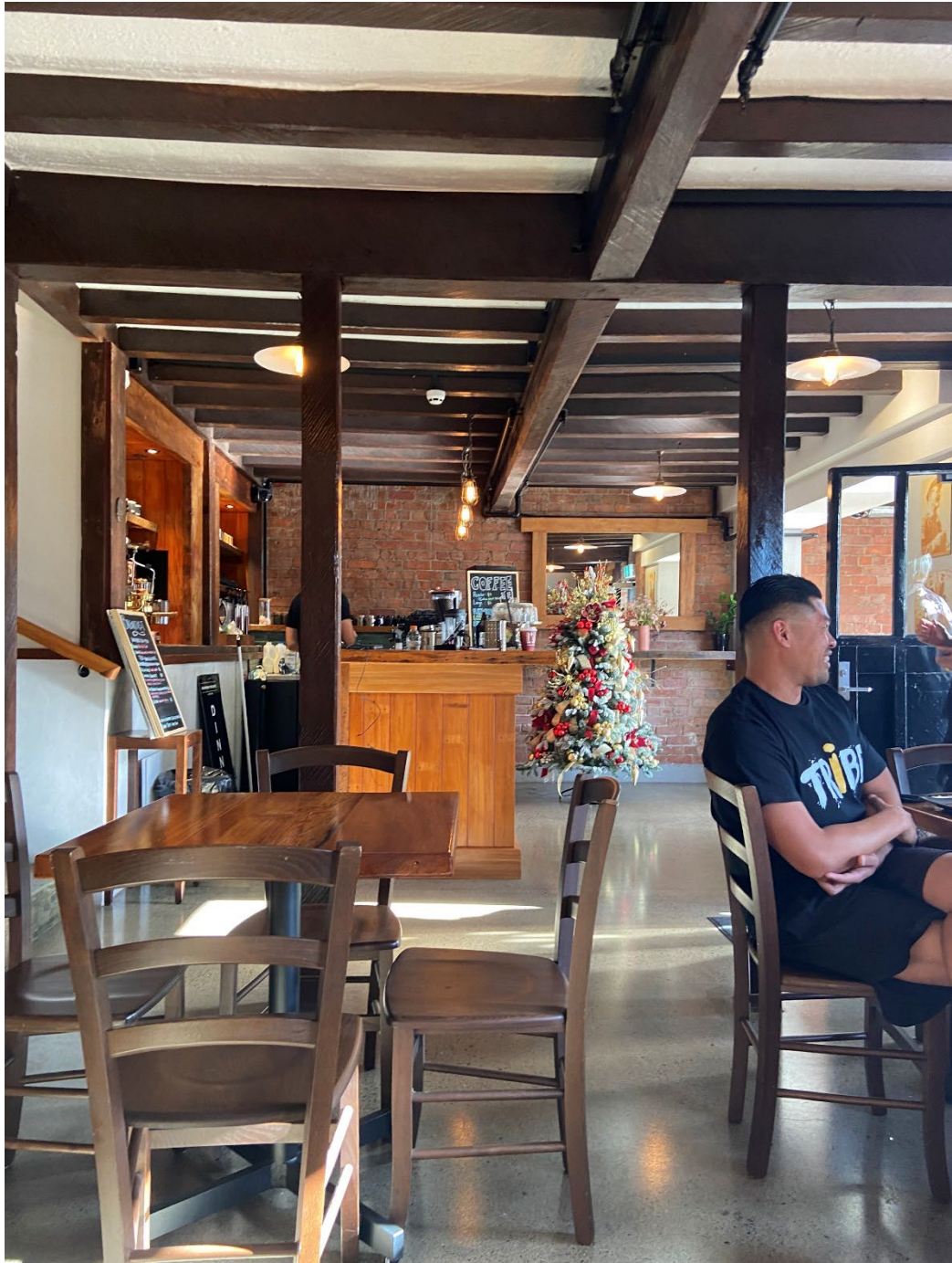
Figure 1: Original jarrah beams and post, ground floor, 2024 41
