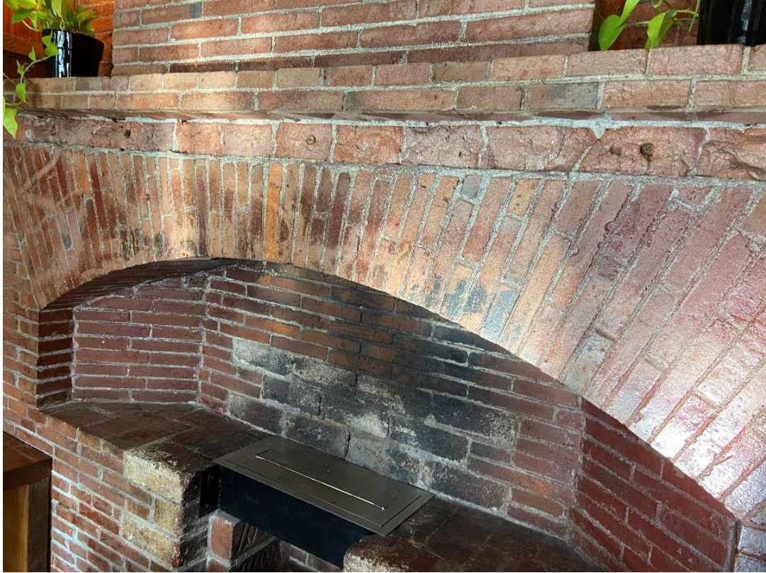
Figure 5: original brick fire place in the inglenook
