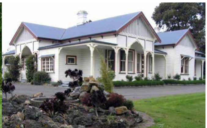
Figure 11: Rangitawa, destroyed by fire and demolished 2015
