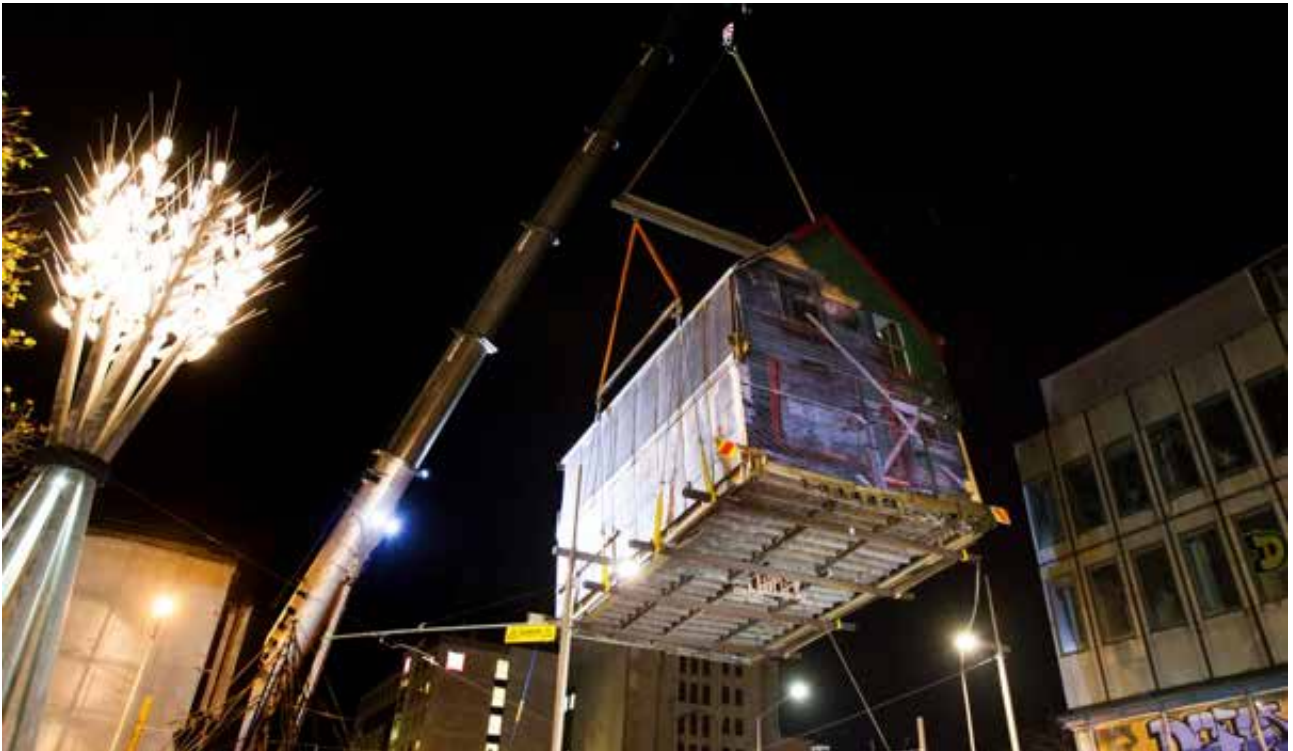
Figure 9: Relocation of Shands Emporium to allow for redevelopment of site after demolition of earthquake damaged buildings
