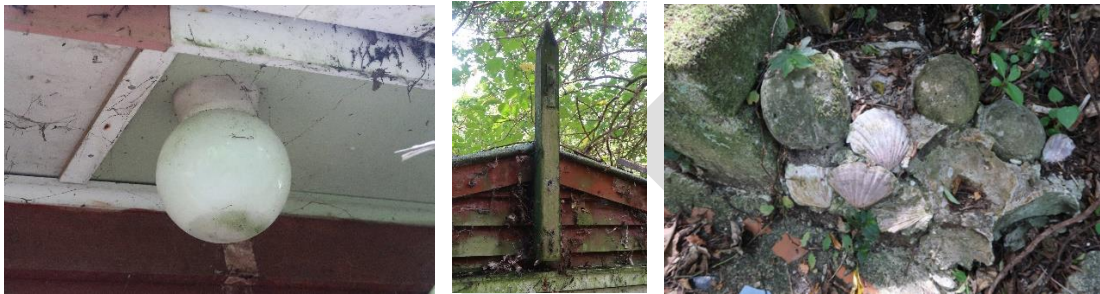
External light (left), finial (centre) and ornamental shellwork beside entrance steps (right)
