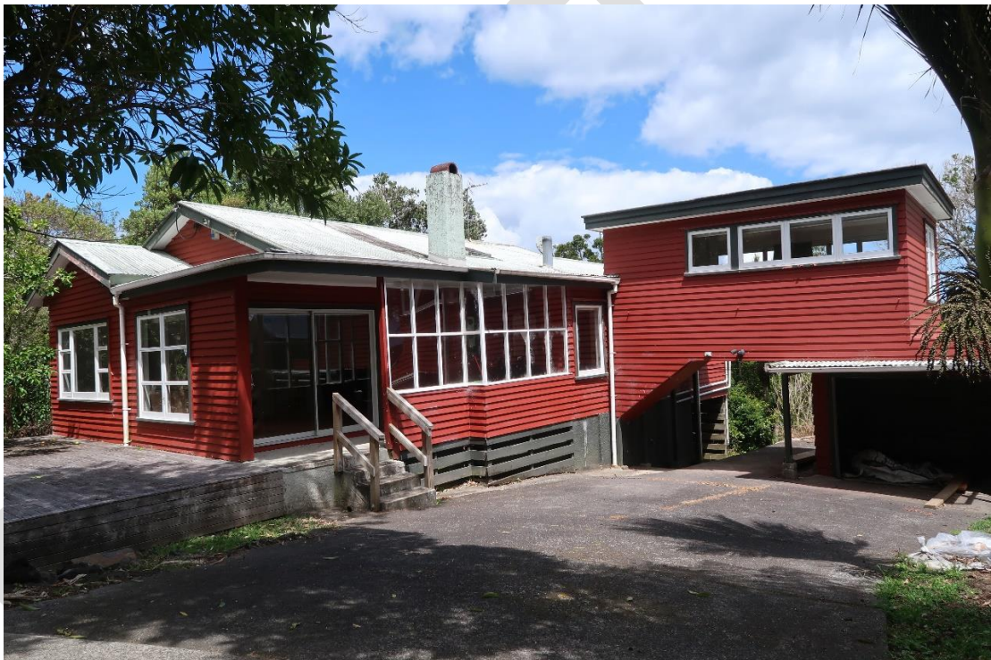
View of house, looking south
