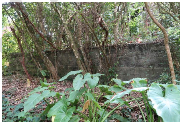
Retaining wall for Shadbolt's vegetable garden, looking north
