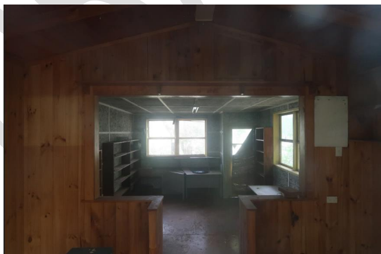
Interior, looking south, showing extension in foreground and main studio behind, including end window with views towards the Waikūmete (Little Muddy Bay) inlet
