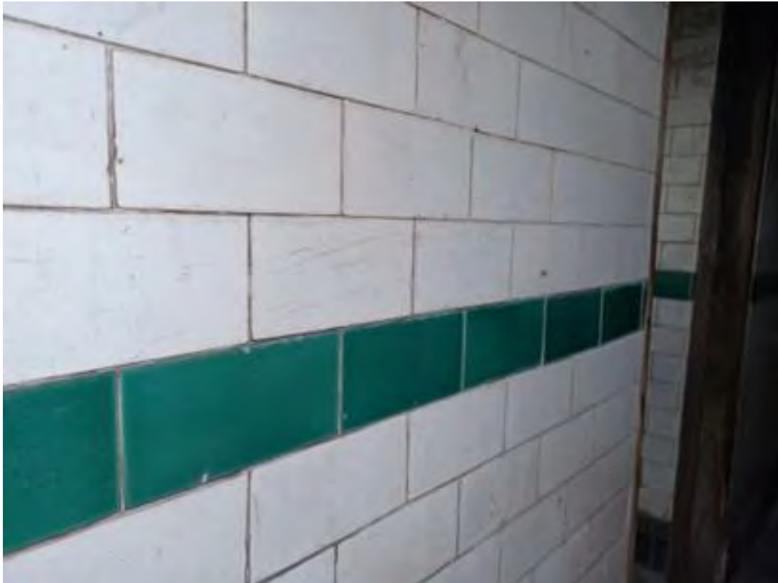
Figure 28: Detail of green tiled dado, Manor Place Convenience 2022, Photograph by Sarah Gallagher, Heritage New Zealand Pouhere Taonga.
