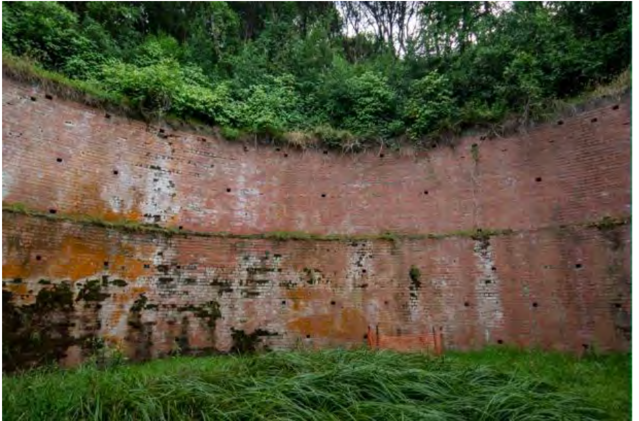
Fig 13: The 10-metre high World War Two Fuel Tank Blast Wall.
