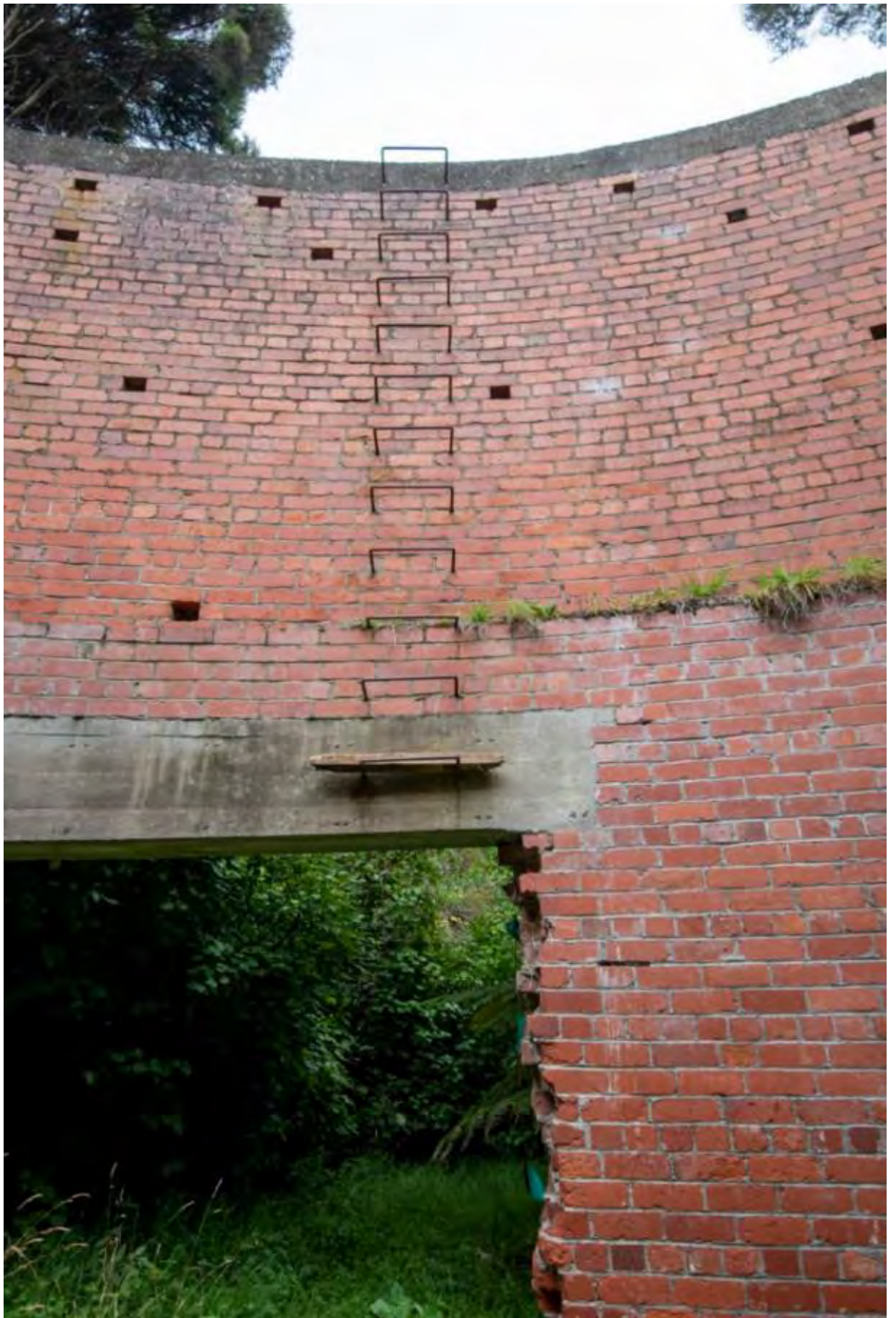
Fig 12: The steel rungs of the access ladder.
