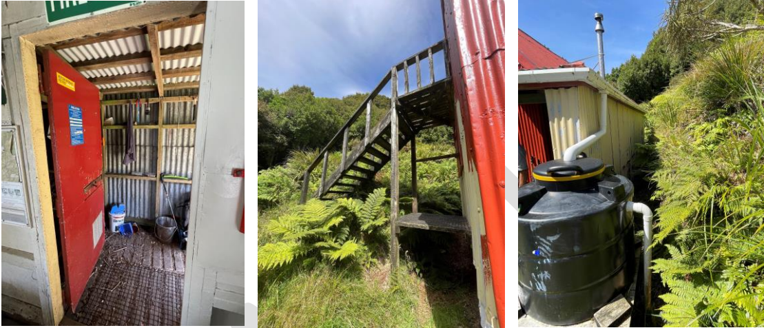
Figure 13: Field Hut's door (left), fire escape (middle), and verandah on the south elevation (right). Natalie Marshall, Heritage New Zealand, 10 March 2024.
