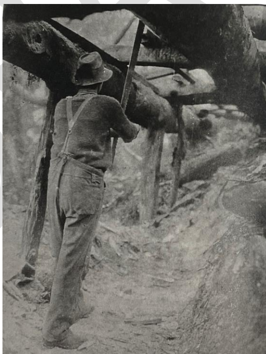
Figure 5: Pit sawing timber for Field Hut, 1924, showing framing being cut from a small, squared length of timber, taken by an unidentified photographer. C Cochran, 'Field Hut Heritage Inventory', p. 6, Collection of Tararua Tramping Club.
