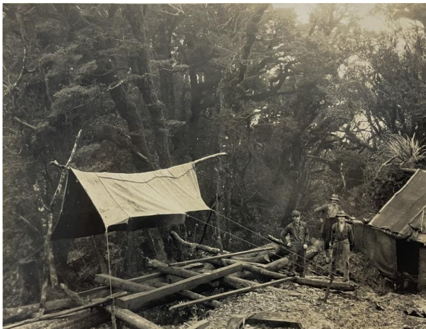
Figure 4: Saw pit used for timber preparation for Field Hut, 1924, showing a canvas fly over the pit, Joe Gibbs (left), and Gibbs' temporary hut with a sacking roof over a timber frame, taken by H C Milne. Album 2, Collection of Tararua Tramping Club.
