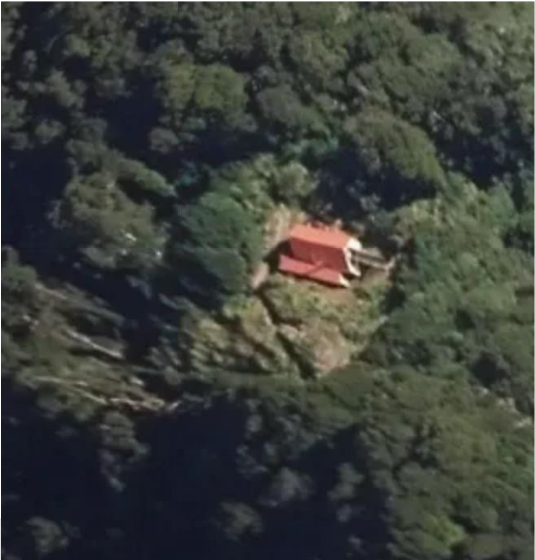
Figure 18: Field Hut is part of Tararua Forest Park. Extent includes part of the land known as Part Ngakaroro 2B Block, Tararua Forest Park ( NZ Gazette 1900 pp.103-104 & NZ Gazette 1967 pp.1551-1553), Wellington Land District, and the structure known as Field Hut.
