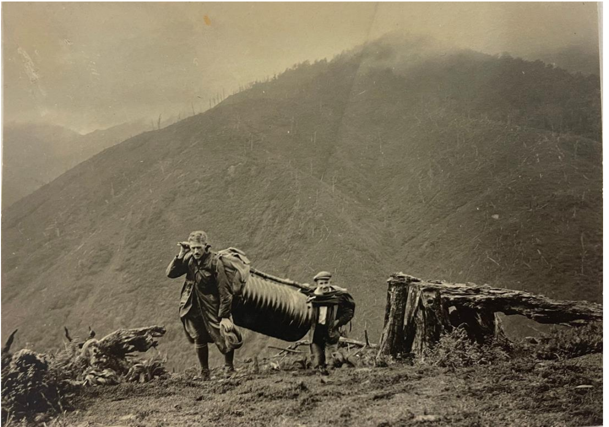
Figure 20: Fred Vosseler (left) and Billy Denton carrying a corrugated iron water tank up to Field Hut, c. 1924, taken by unidentified photographer. Album 2, Collection of Tararua Tramping Club.
