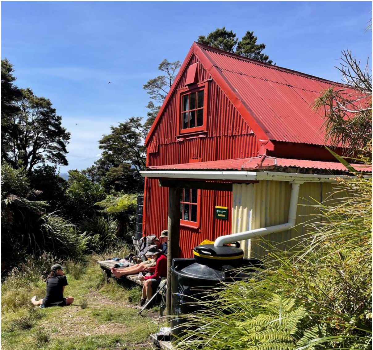
Field Hut, west elevation, Tararua Forest Park. Natalie Marshall, Heritage New Zealand, 10 March 2024
