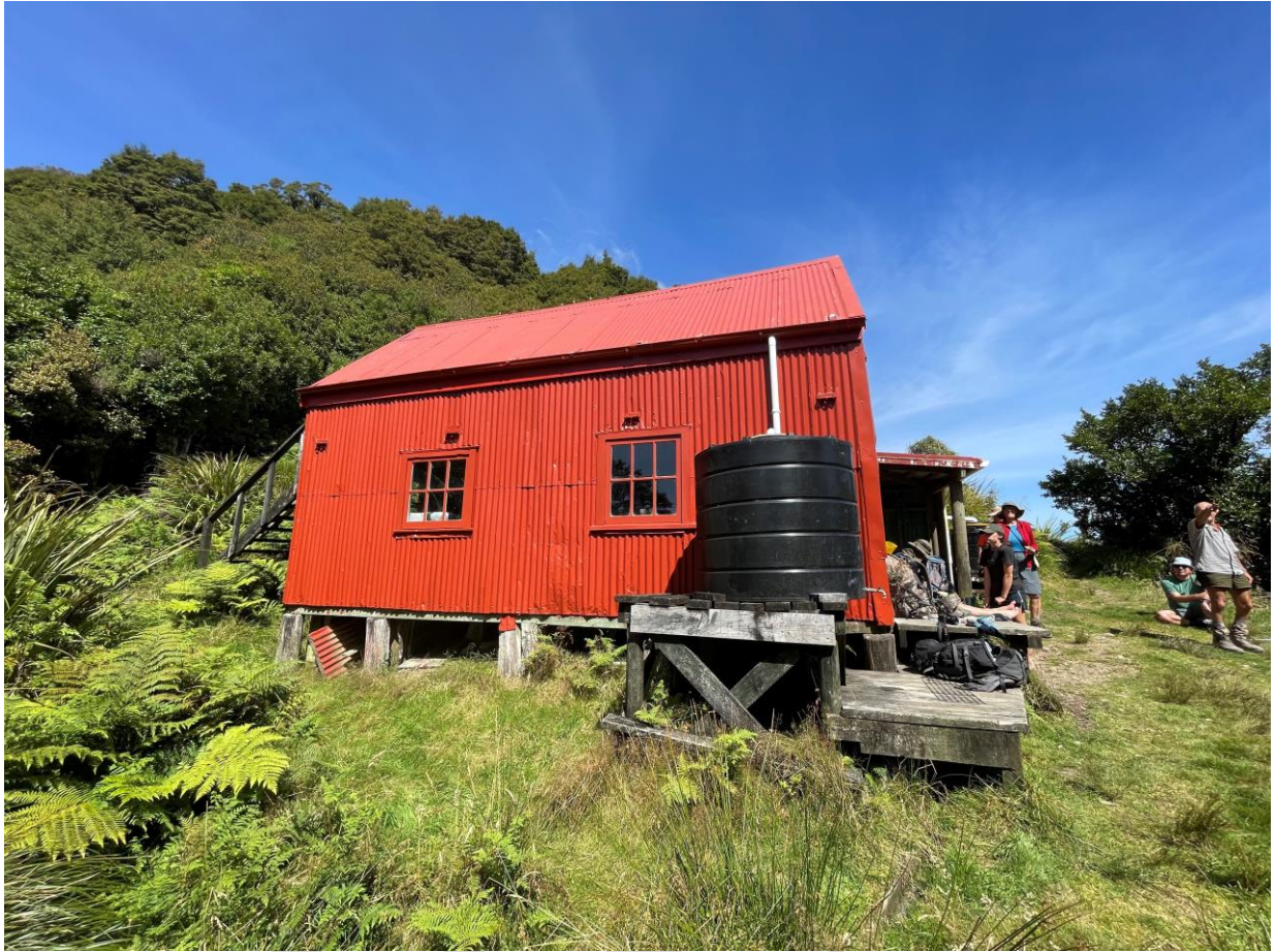
Figure 27: Field Hut, north elevation. Natalie Marshall, Heritage New Zealand, 10 March 2024.
