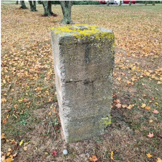
Figure 14 Concrete pier, R. Burgess 12 Apr. 2024, Heritage New Zealand Pouhere Taonga
