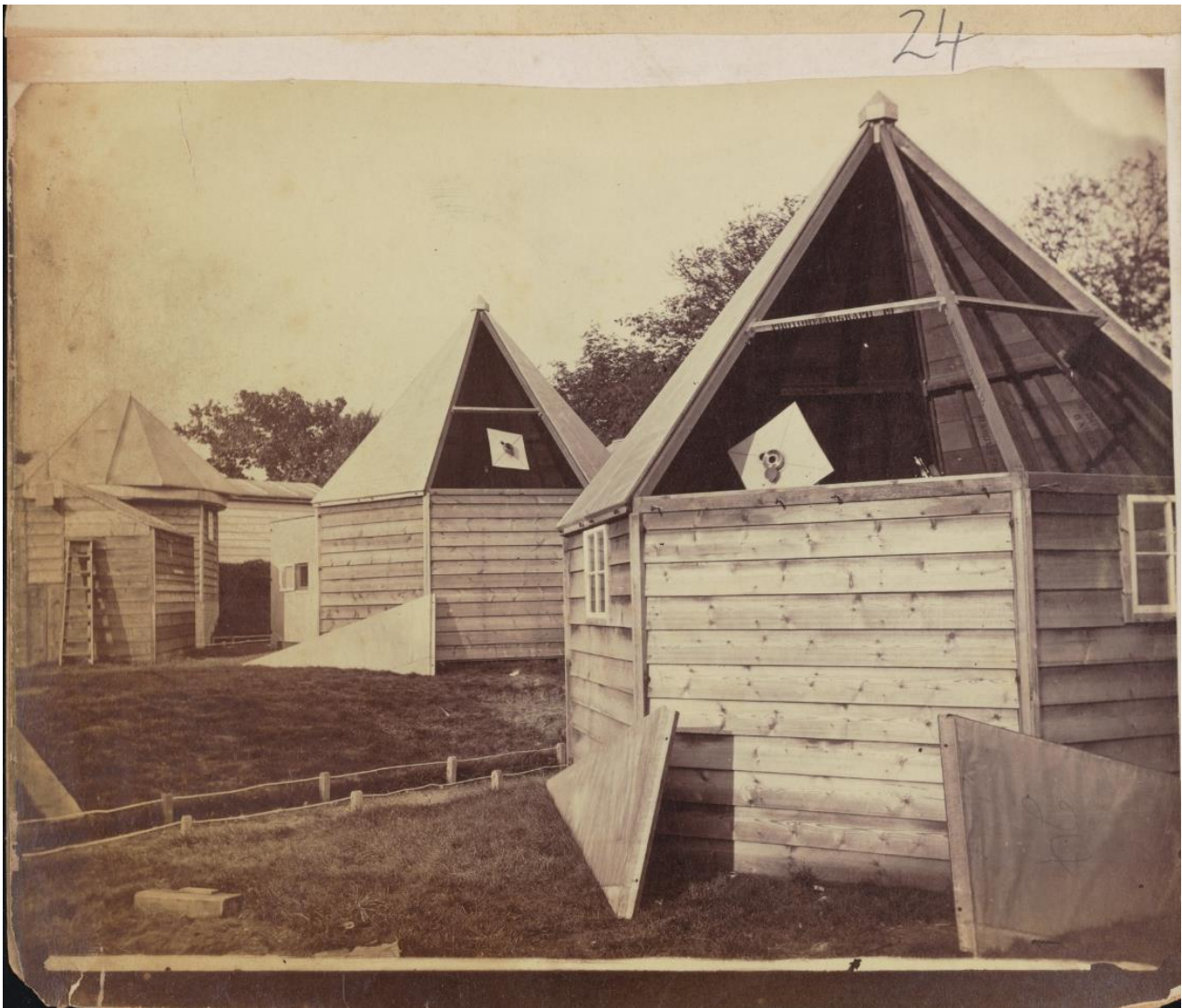
Figure 6 Photograph showing various observing huts with their roofs opened, Greenwich (Cambridge University Library, RGO 6/276: 24). These huts are at the Greenwich hut in England before their despatch to their intended observation stations around the world. The closest hut (right) is stencilled 'Photoheliograph' and 'Station D', showing that this is one of the huts subsequently brought out to New Zealand and reassembled at Burnham. (Copyright Cambridge University Library, Licensed under Creative Commons Attribution – Non-Commercial).
