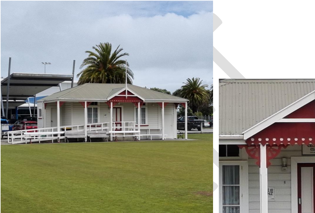
Pavilion showing north front and east side elevations (left), and detail of verandah fretwork and gable valance (right), R. Burgess, 29 Nov. 2023, Heritage New Zealand Pouhere Taonga
