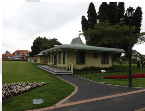
Rotorua Government Gardens Croquet Pavilion, Dec. 2014, R. Burgess, Heritage New Zealand Pouhere Taonga
