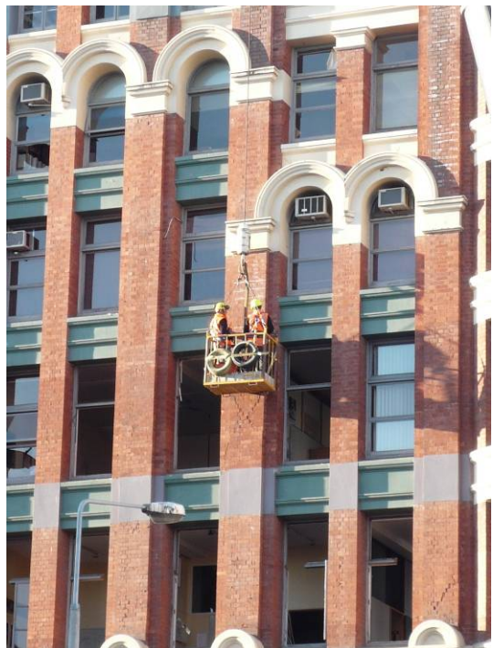
Manchester Courts showing inspection of diagonal cracking on façade after earthquake of 4 September 2010 (Malcolm Duff, 26 September 2010, NZHPT)
