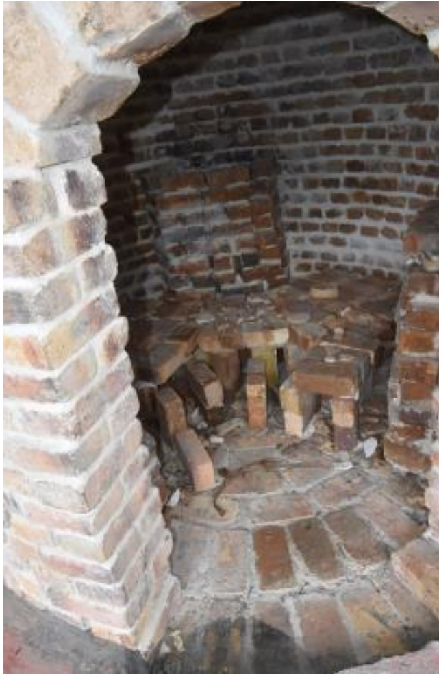
Figure 2. The interior of the easternmost kiln with a shelf for placing pottery on. Constructed 1971.
