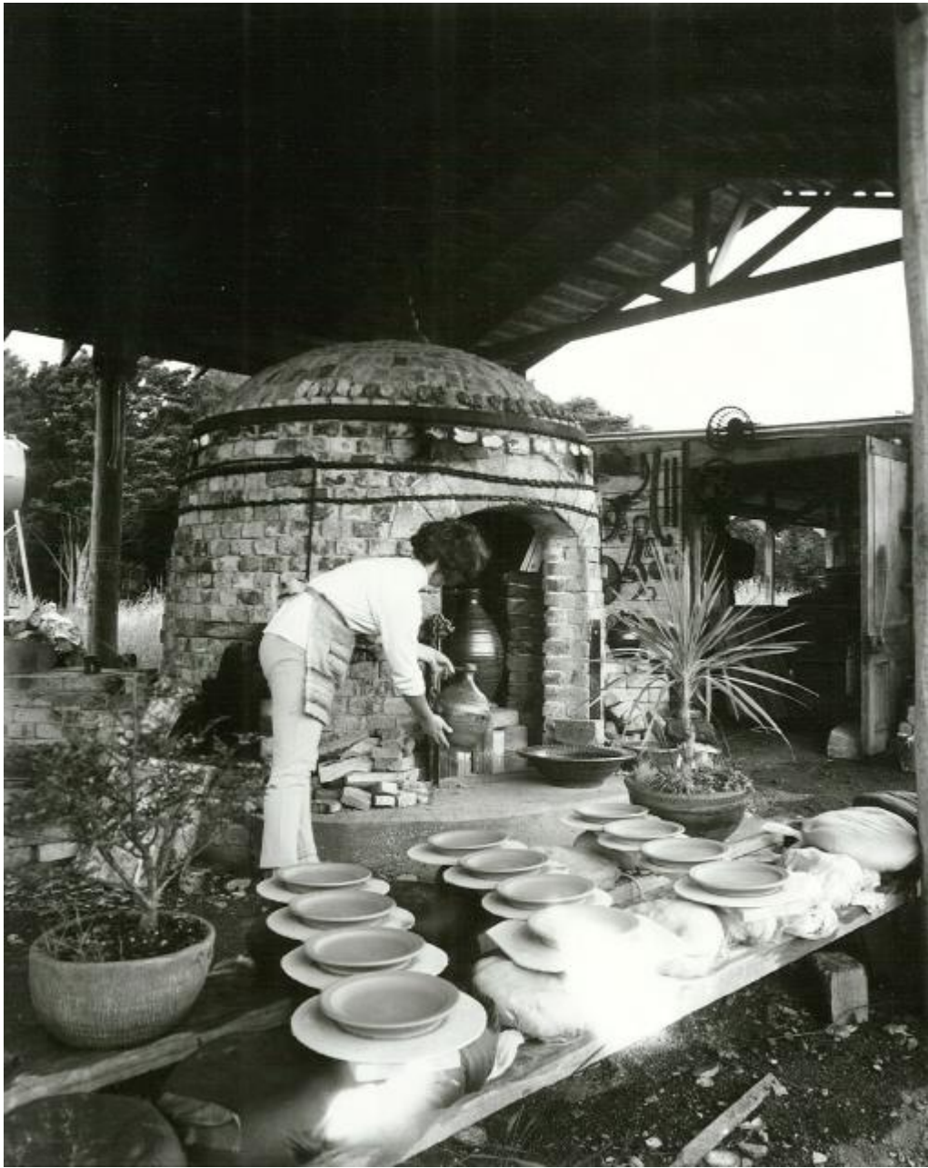
Figure 13. The easternmost glost kiln in use. Photographer: Cleal, Archives New Zealand – Communicate New Zealand Collection, R24808117, 1973-1973, Box Number B2910, Creative Commons BY2.0 license.
