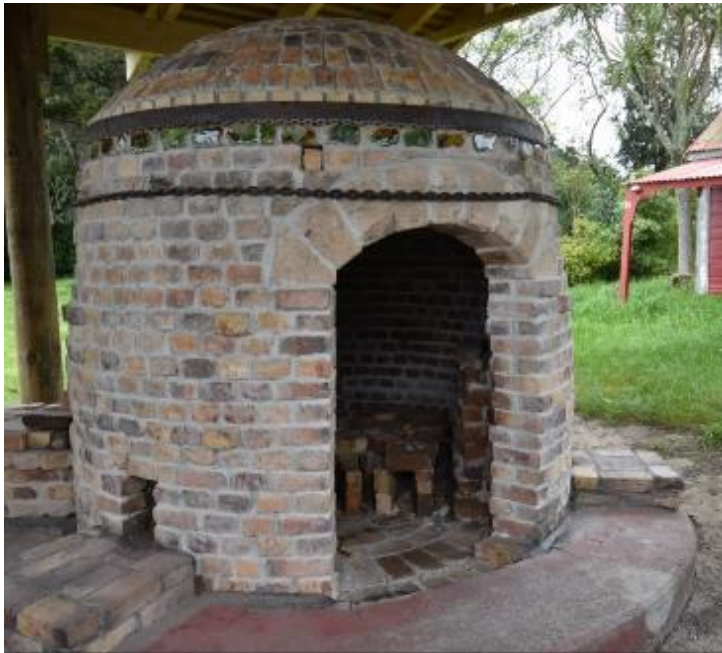
Figure 1. The top of the eastern kiln, with chain strapping and metal band. Constructed 1971.
