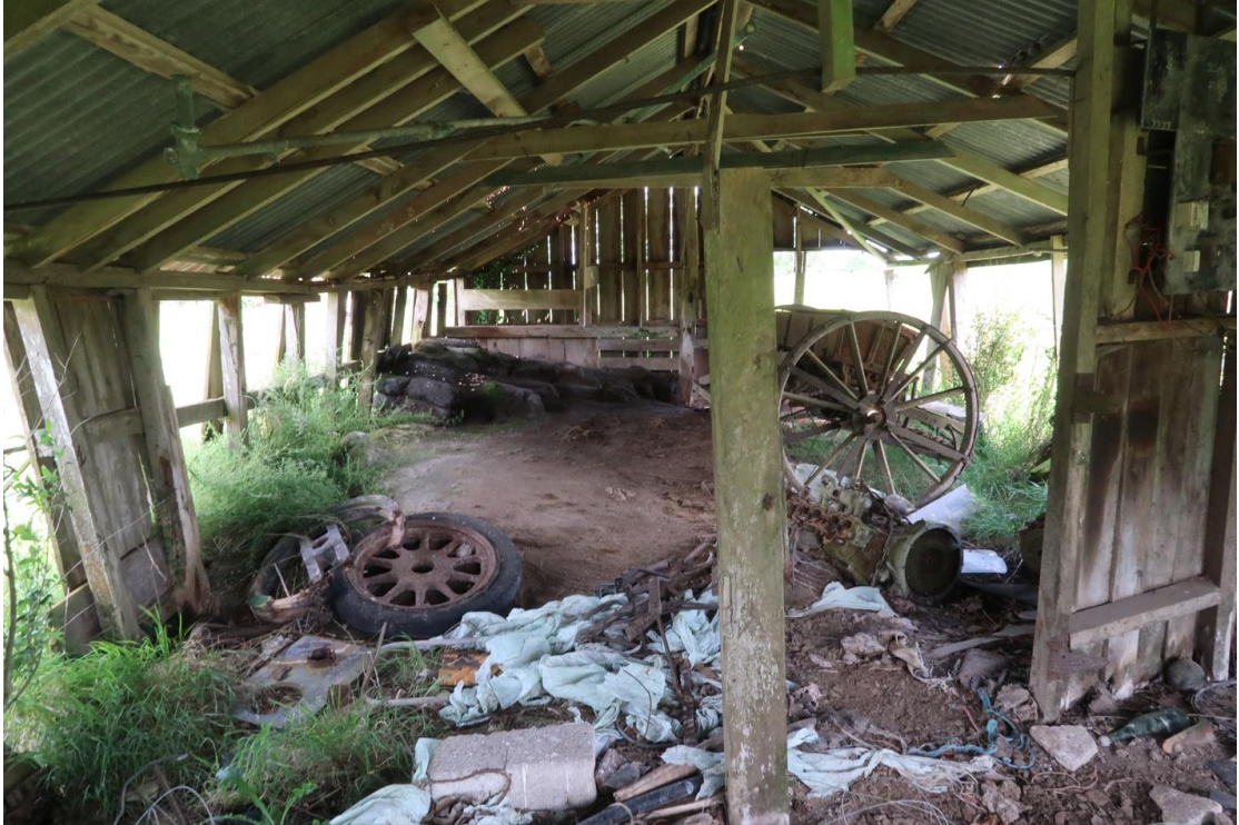
Main internal space, with separating room at right, looking south
