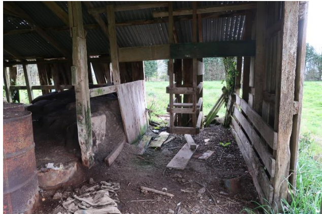
Milking bails at south end of main space, looking east
