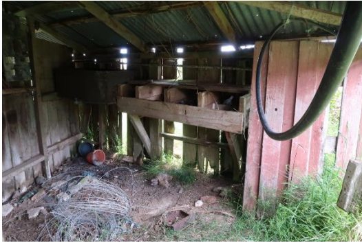
Separating room, looking southwest
