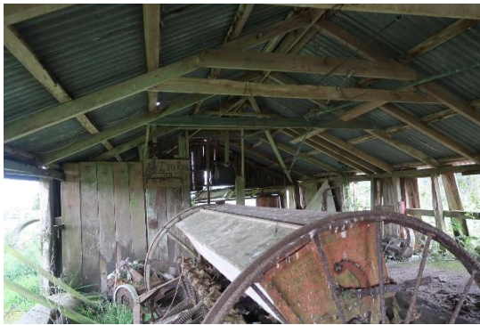
Cowshed interior with roof framing, looking north
