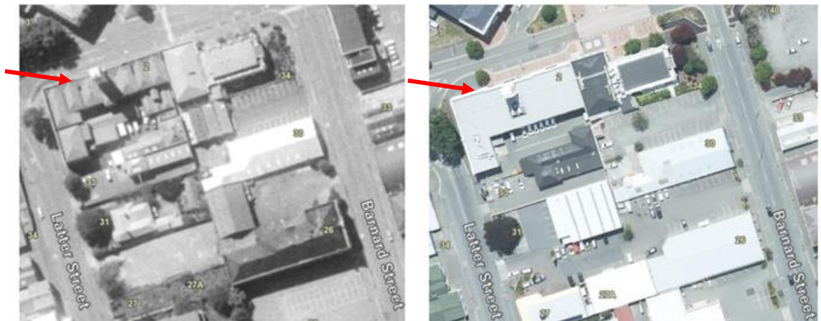
Aerial photographs showing Timaru City Council Offices and Former Public Library rooflines in the 1980s compared to current flatter profile in the photograph dated circa 2020.
