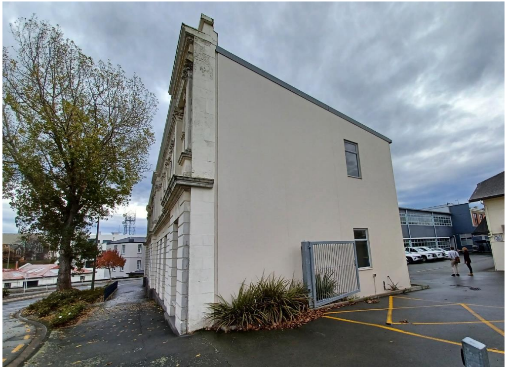
View from south-west showing original west elevation façade and modern south facades from the 2000s redevelopment, R. Burgess, 9 May 2023, Heritage New Zealand Pouhere Taonga
