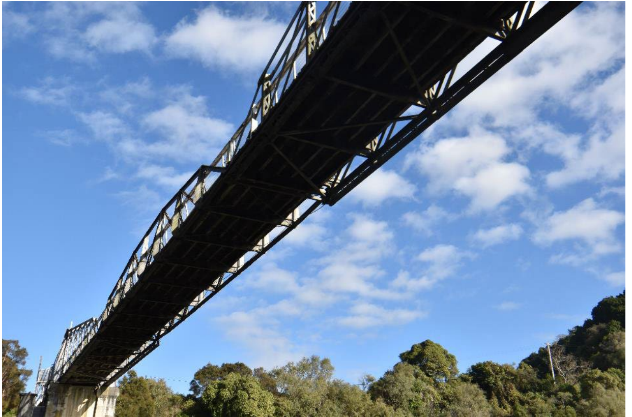
Figure 14: Underside of the deck of Mangaweka Cantilever Bridge
