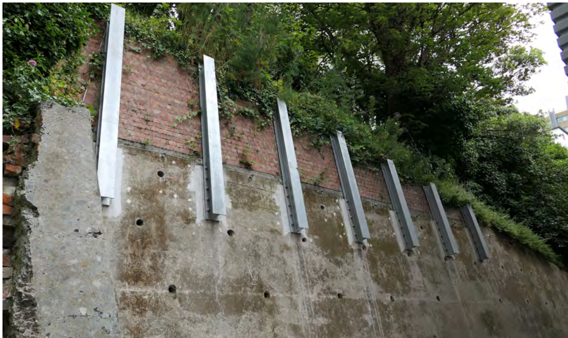
2018 securing work to the brick wall on top of the west retaining wall.
