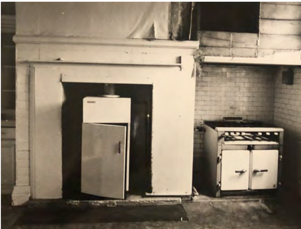
Kitchen before restoration, 1980, HNZPT Collection
