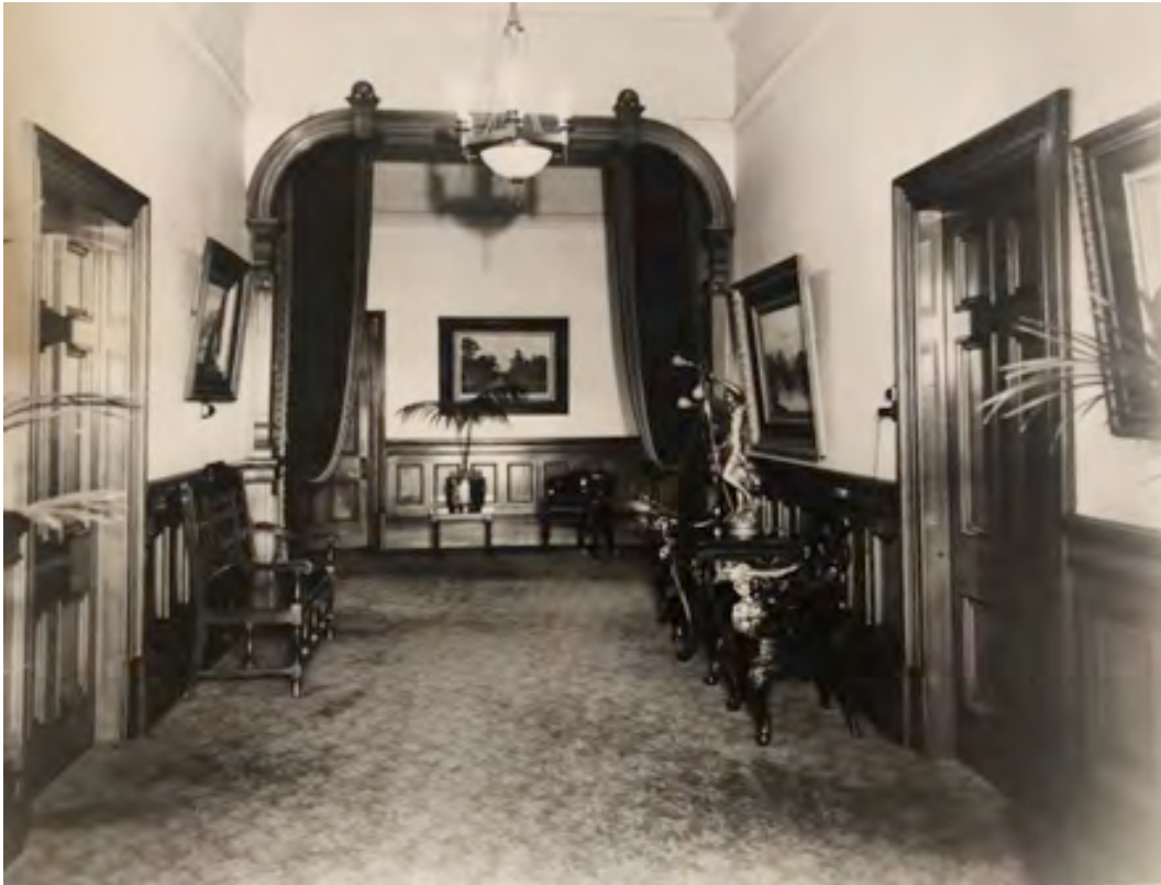
The ground floor repaired after the fire – front hallway, 1947, HNZPT collection
