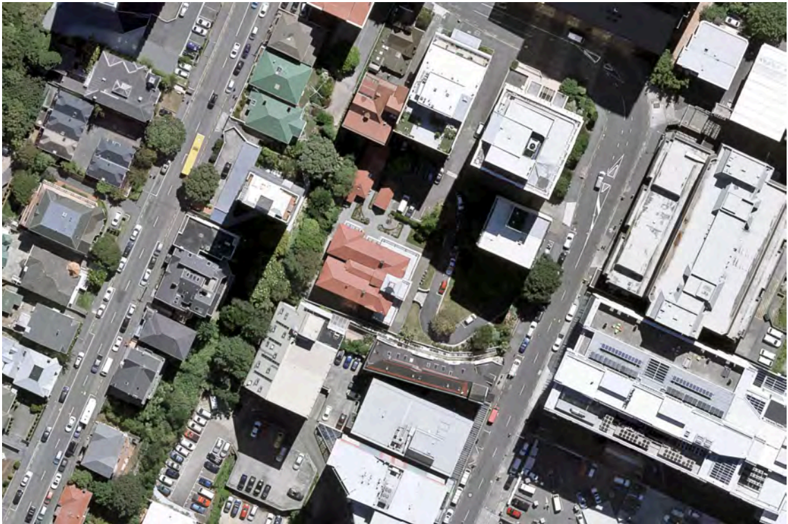
Aerial view of Antrim House and its immediate setting. (Image from Wellington Maps, 2020)
