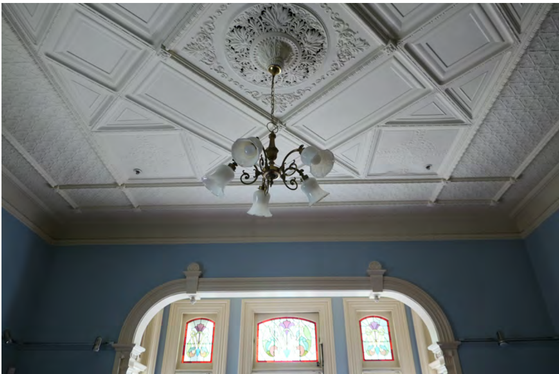
Sitting Room ceiling
