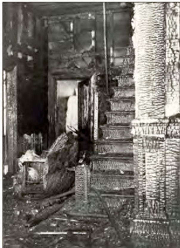
The remains of the tower staircase after the fire, 1940
