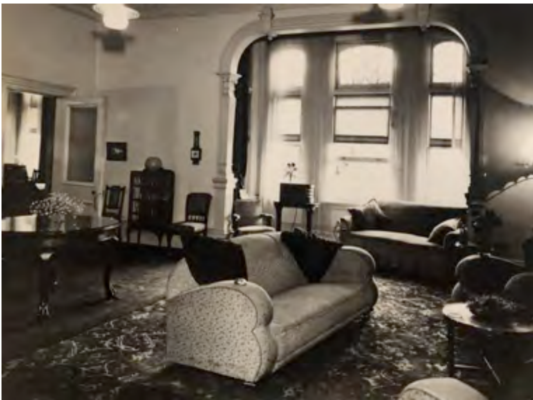
The ground floor after the fire – the Hickson's sitting room [former Dining Room, now Records Room/Reception], 1947, HNZPT Collection.
