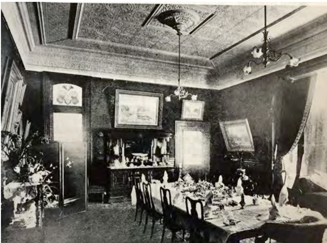
The Hannah's dining room (now Records Room/Reception), 1906. Briscoe's catalogue c1907, taken from Attwell, p31. Note the door to the billiard room on the right, and the window topped with a leadlight that was made internal by the addition of the billiard room [the window was later removed]
