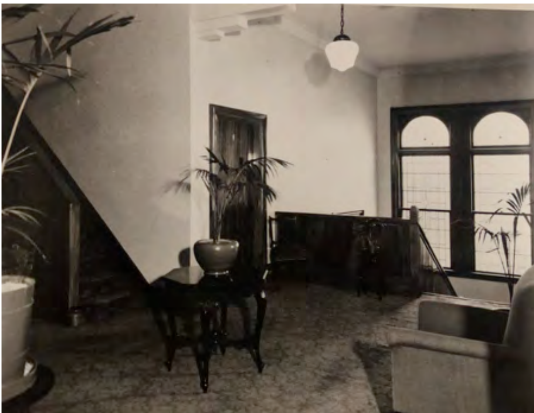
Top of the stairs as repaired after the fire, 1948/49. Note the two staircases, now with solid balustrades, and the Art Deco-style ceiling cornice. HNZPT Collection
