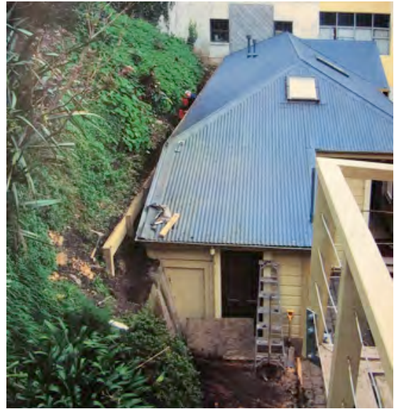
Work to build a new retaining edge and drain to intercept surface water from the top of the bank at the stables, 2005. HNZPT file.
