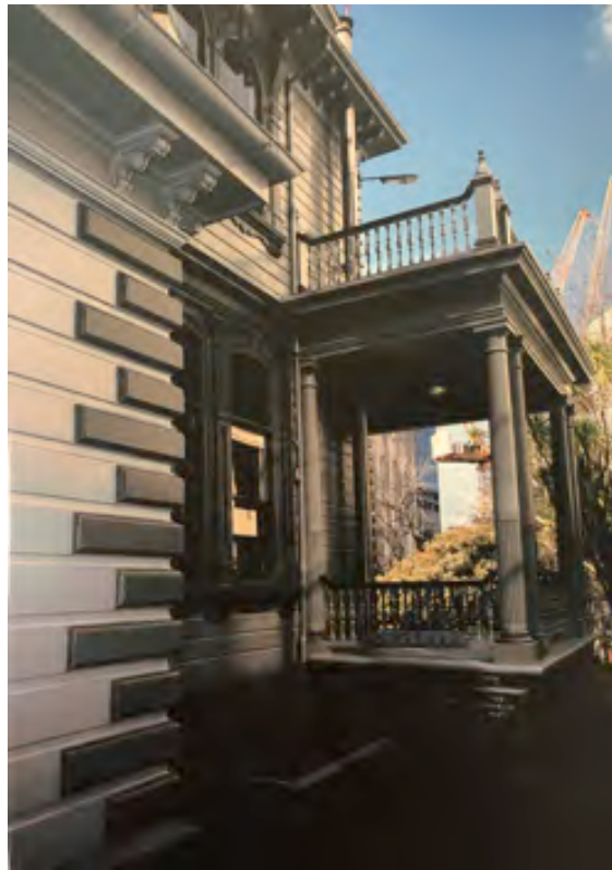
Before and after the removal of the fire escapes on the southern façade, and reinstatement of missing balustrades and repainting, in 2009. HNZPT Collection
