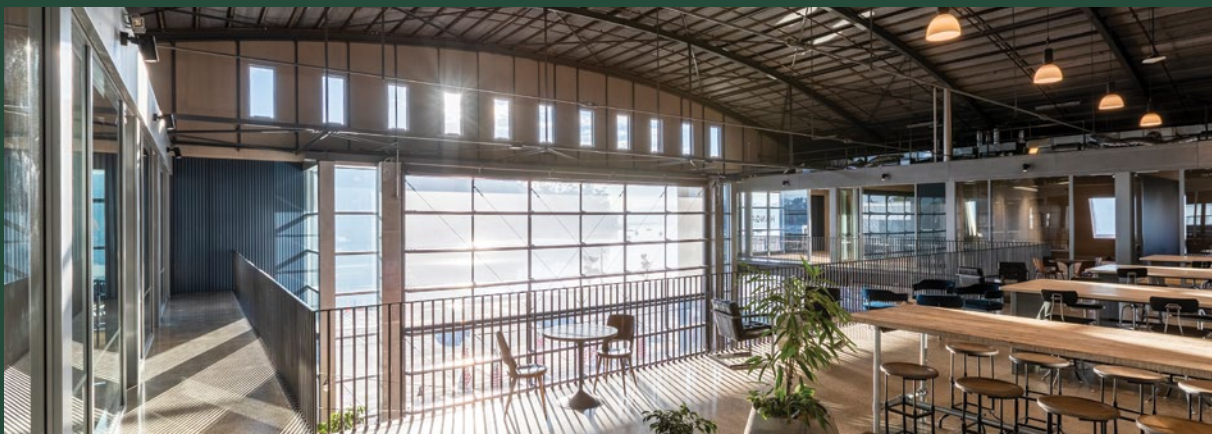
The Sunderland Hangar has been adaptively reused to serve a mix of purposes for local residents.
