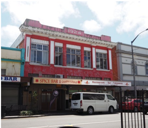
Before and after photos of 88 Guyton Street, supported by the Whanganui Heritage Fund.
