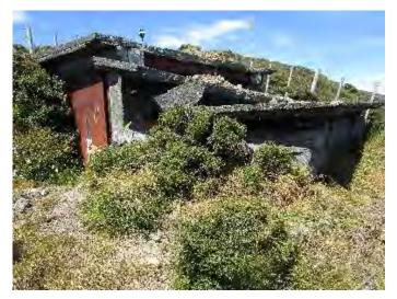
The observation post for the Palmer Head Battery is built into the slope and constructed of reinforced concrete. This building retains part of its camouflage (a layer of earth and vegetation directly on its roof) but the cantilevered roof over the viewing slit has collapsed,
