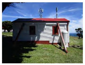
The exterior of the lapped weatherboard-clad timber garage has been fully renovated and a new roller door installed. This small structure is exposed to southerly gales and was braced by timber buttresses on the north elevation 1968 following the devastating Cyclone Giselle
