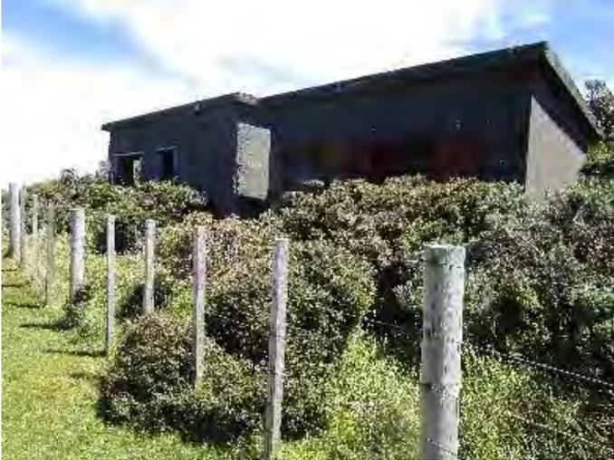
On the north side of the hill below the observation post is the former barracks (later the wireless room; left) for the observation post. Also built of reinforced concrete, this building is rendered on the outside. Alongside it is another building – probably the engine room – constructed during the war but not rendered. Both buildings are flat roof, rectangular boxes and are largely reduced to shells. The concrete water tank that services the barracks is directly above these buildings.
