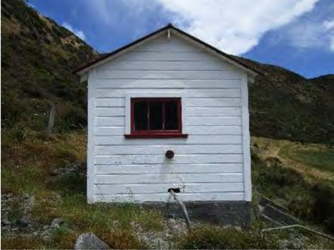
The pumphouse is a small timber building clad in rusticated weatherboards and a corrugated iron roof resting on concrete foundations. The interior is unlined, and the timber is weathered and watermarked. The concrete base of the pump, which has been removed, remains in place.
