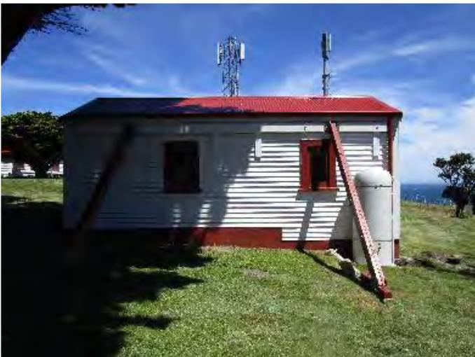
The exterior of the lapped weatherboard-clad timber garage has been fully renovated and a new roller door installed. This small structure is exposed to southerly gales and was braced by timber buttresses on the north elevation 1968 following the devastating Cyclone Giselle
