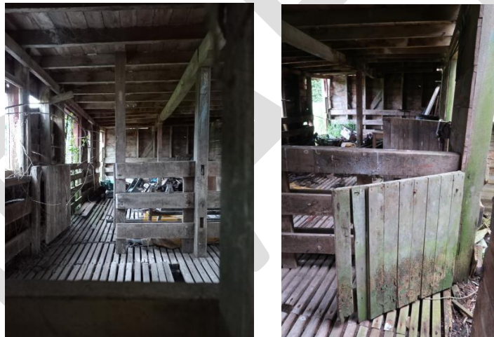
Internal pens at west end of initial structure after conversion to a woolshed, looking east (left) and door from internal pen to catching pen in south lean-to, looking northeast (right)
