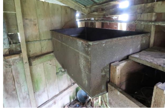
Metal tank in separating room, looking southwest
