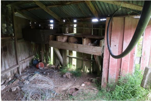
Separating room, looking southwest
