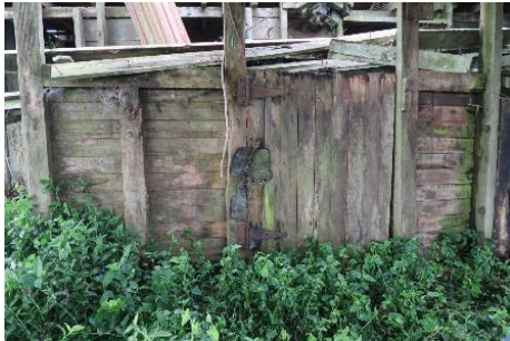
Catching pen in south lean-to, with door
