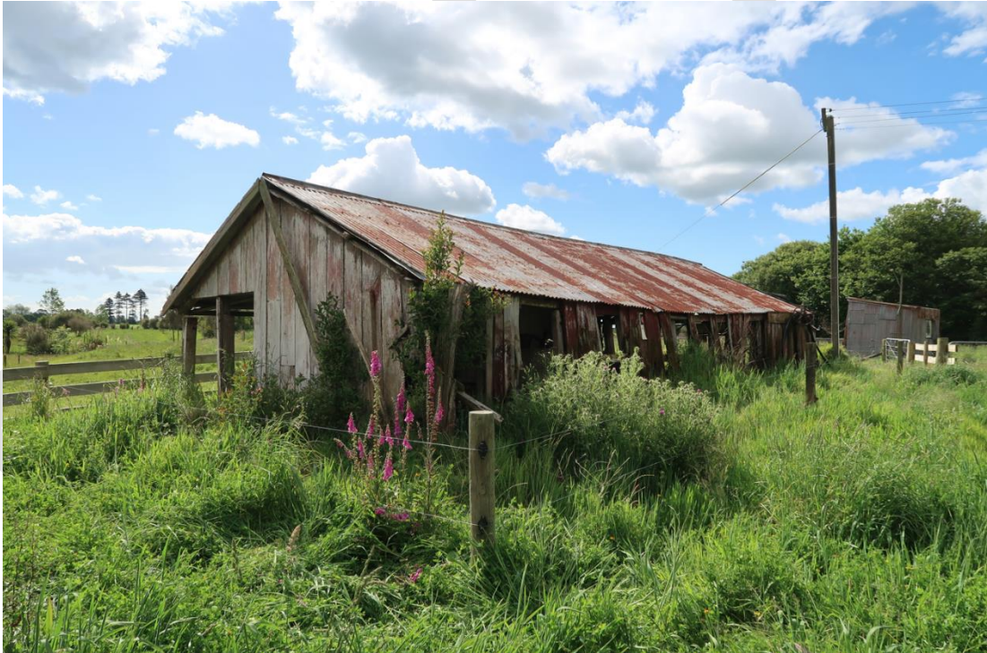
Cowshed, looking northwest with whare in background
