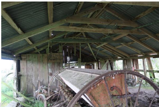
Cowshed interior with roof framing, looking north
