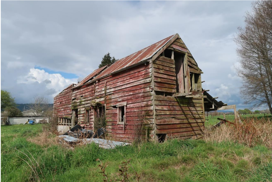
Woolshed (including former stables), looking southeast
