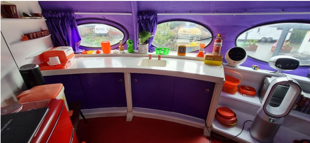
Kitchen area showing original fibreglass moulded bench, sink, cupboards and shelves (R. Burgess, 23 June 2023, Heritage New Zealand Pouhere Taonga)
