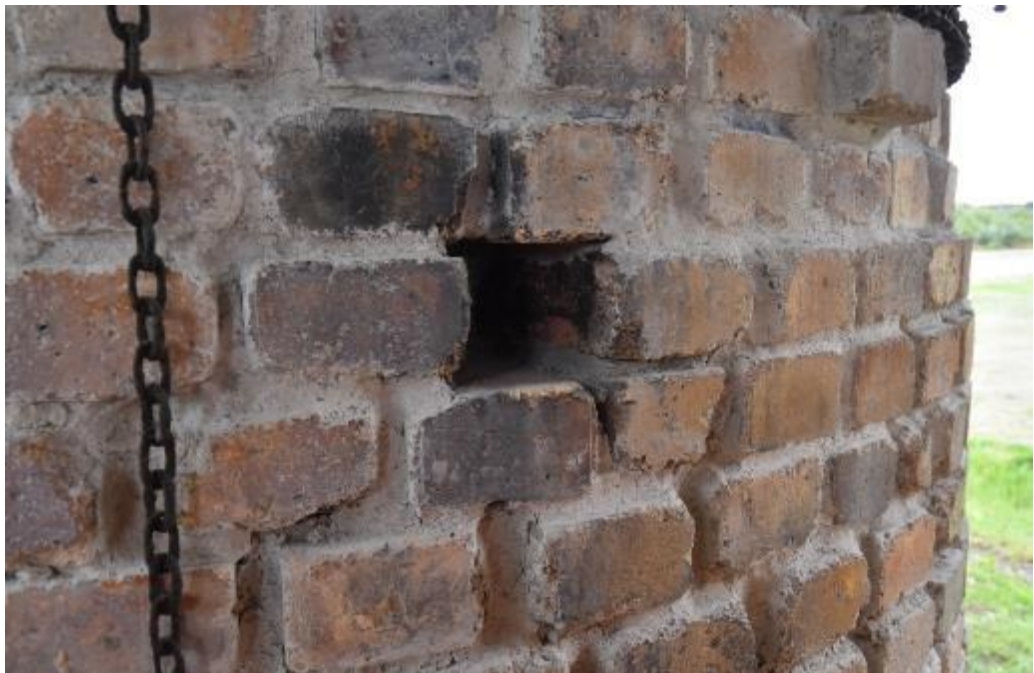
Figure 4. The hole through which salt was thrown to create salt glazing. Constructed 1971.
