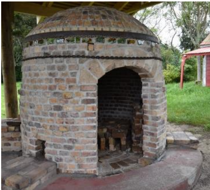
Figure 1. The top of the eastern kiln, with chain strapping and metal band. Constructed 1970.
