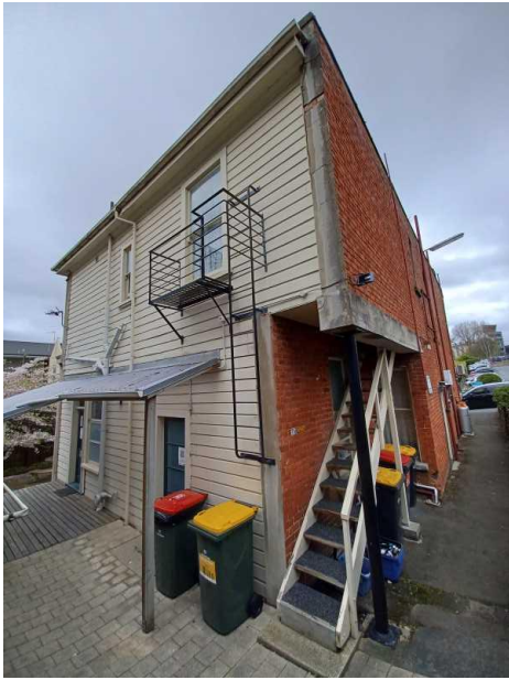
Figure 8: View from the north showing the rear elevation clad in weather board, and the rear stairs that provide access to the flats upstairs.
