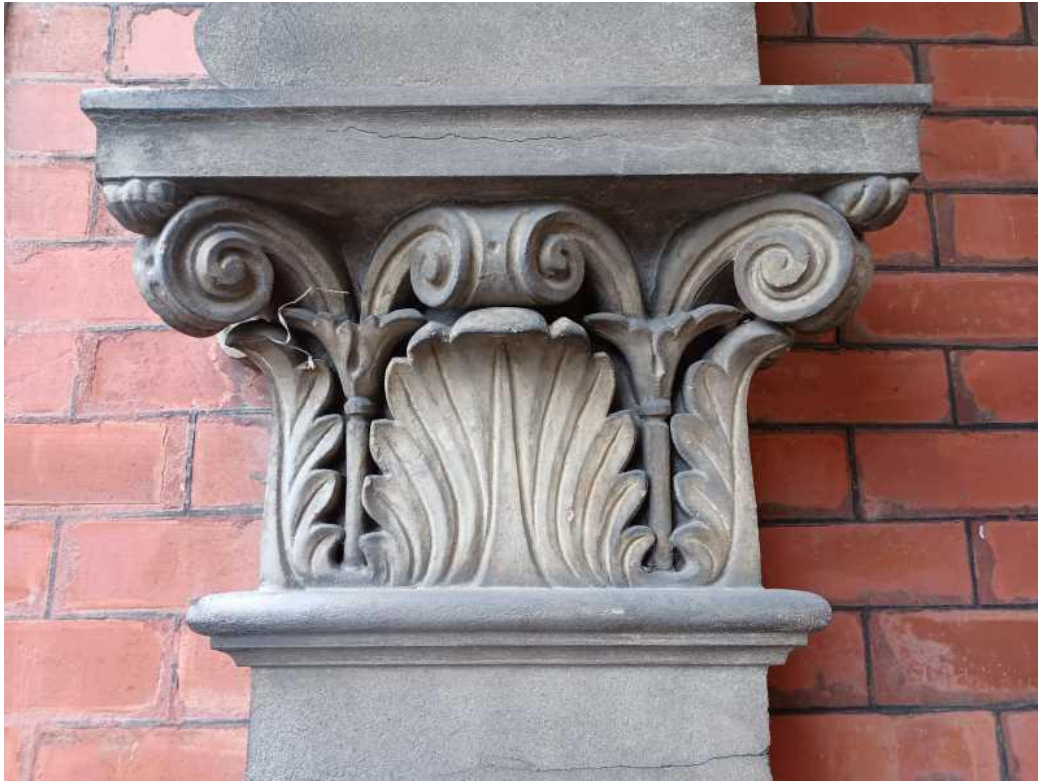
Figure 6: Detail of one of the Corinthian capitals and red mortar with black tuck pointing. Sarah Gallagher, Heritage New Zealand Pouhere Taonga, 10 October 2022.
