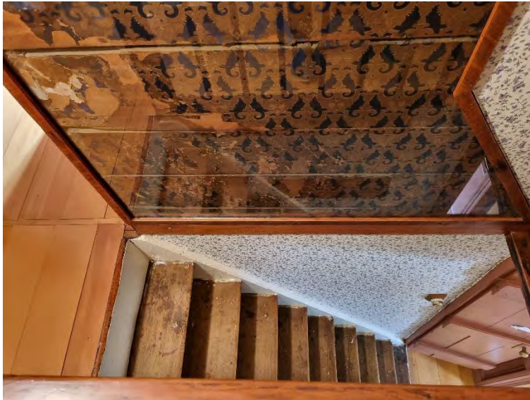
Figure 21. View from first floor landing looking back down the narrow staircase, and showing early wallpaper with protective glazing (Robyn Burgess, 20 December 2022, Heritage New Zealand Pouhere Taonga) [Note lining board behind the wallpaper which shows circular sawn kahikatea, attached with sheet-sliced nails as found throughout the rest of the house]. 120
