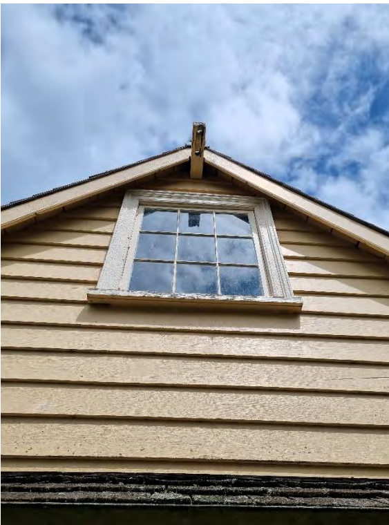
Figure 18. Detail showing pulley above gable window (east elevation), Robyn Burgess, 20 December 2022, Heritage New Zealand Pouhere Taonga
