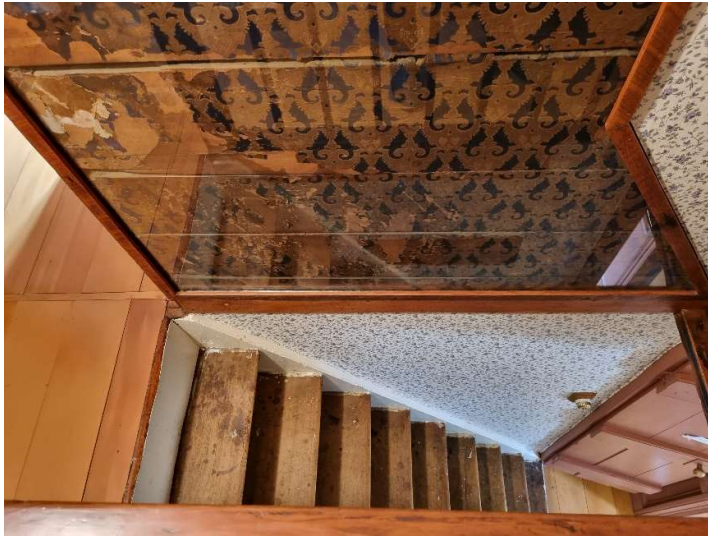
Figure 12. View from first floor landing looking back down the narrow staircase, and showing early wallpaper with protective glazing (Robyn Burgess, 20 December 2022, Heritage New Zealand Pouhere Taonga) [Note lining board behind the wallpaper which shows circular sawn kahikatea, attached with sheet-sliced nails as found throughout the rest of the house]. 115
