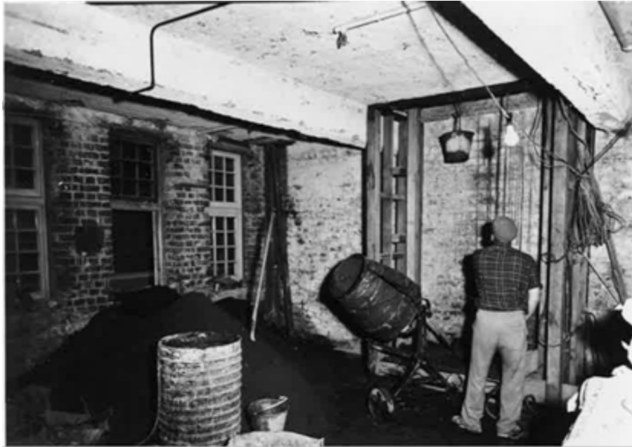
Remedial work under way, 1956. Image taken in one of the stack rooms. Note the walls taken back to the brick, and the timber-framed shaft for the book lift. (10932½, ATL)
