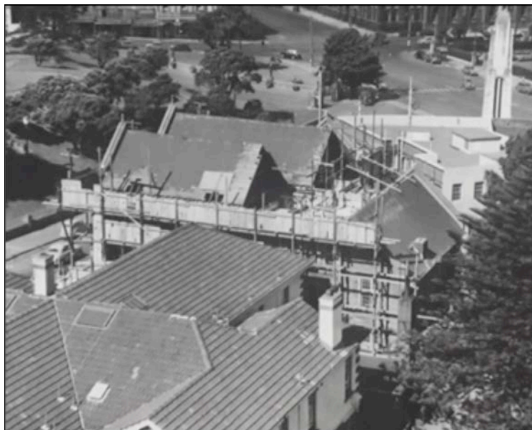
Structural strengthening of the library under way, with Bowen Hospital in the foreground. The fourth floor stack room and concrete “dome” has been removed and the roof is open. November 1955. (EP/1955/2469-F, ATL)
