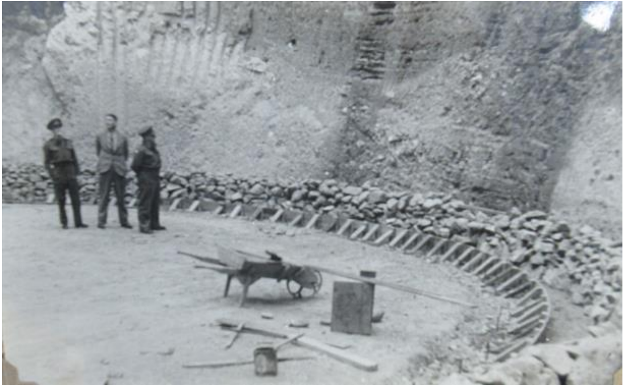
Fig 8: AR17 under construction, 18 December 1942: the excavation is complete and work on the foundation has commenced. 'Defence Works and Buildings – Air Department Royal New Zealand Air Force [RNZAF] bulk fuel storage – Site AR17 – Paekakariki 1942-1942', Item ID R21064922, box 796, file 23/553/17, Public Works Department (ACHL), Archives New Zealand
