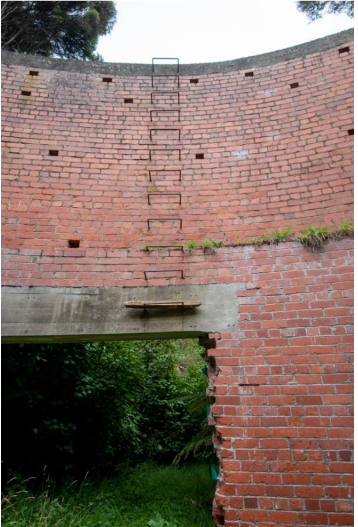
Fig 12: The steel rungs of the access ladder.
